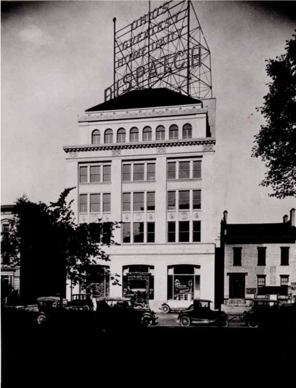
The YMCA building was demolished in 1923, and the Columbus Dispatch building took its place. The Andrews house to its right was razed in January 1927. ( Columbus Dispatch )
